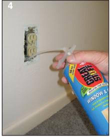
Figure 3. The air gaps and holes around fixtures like this light switch all leak sound. Seal them!
