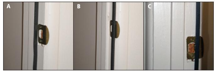
Figure 7. Install gasketing so that it's compressed by the door when you close it (A). Don't put it along the edge where the striker plate goes (B and C); it may seal tightly at first, but as you use the door, friction will cause it to eventually get torn loose.
