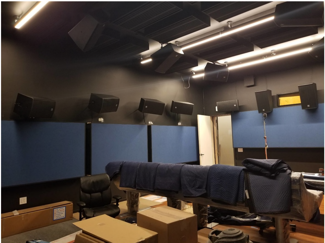
Closing in on completion—rear view.
