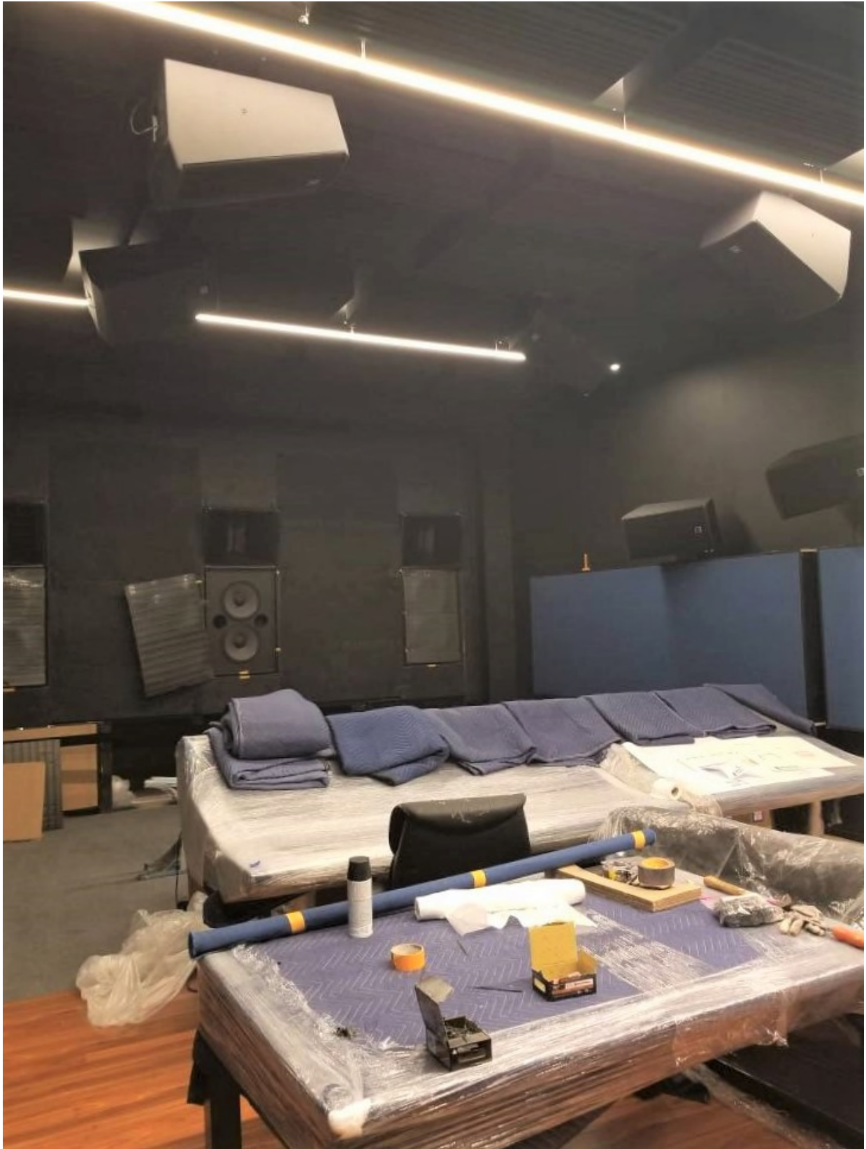
Closing in on completion—front view.
